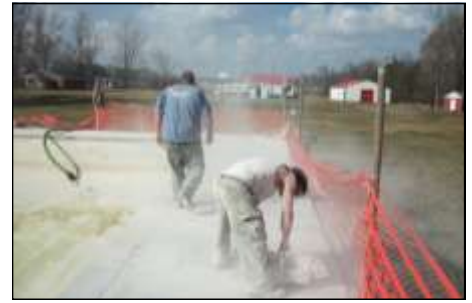
Removal of fence, deck and Old plumbing in March
