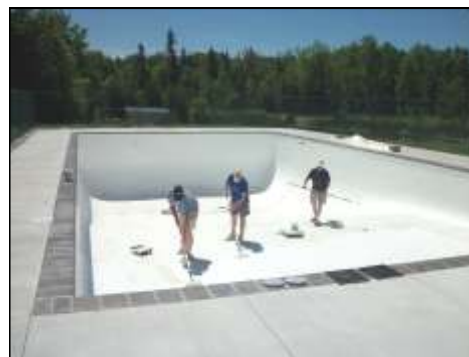
Our volunteers applying the coats of rubberized paint to the pool surface
