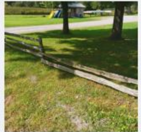
Old cedar fencing
